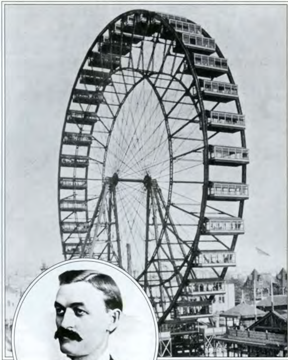
George Ferris (left) caused a sensation in 1893 with his Nevada-inspired wheel. It was 250 feet in diameter and could hold 1,440 passengers. A two-revolution ride lasted 20 minutes.
