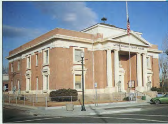
The 1912 Lyon County Courthouse, designed by Frederick J. DeLongchamps, offers architectural interest on Yerington's Main Street.
