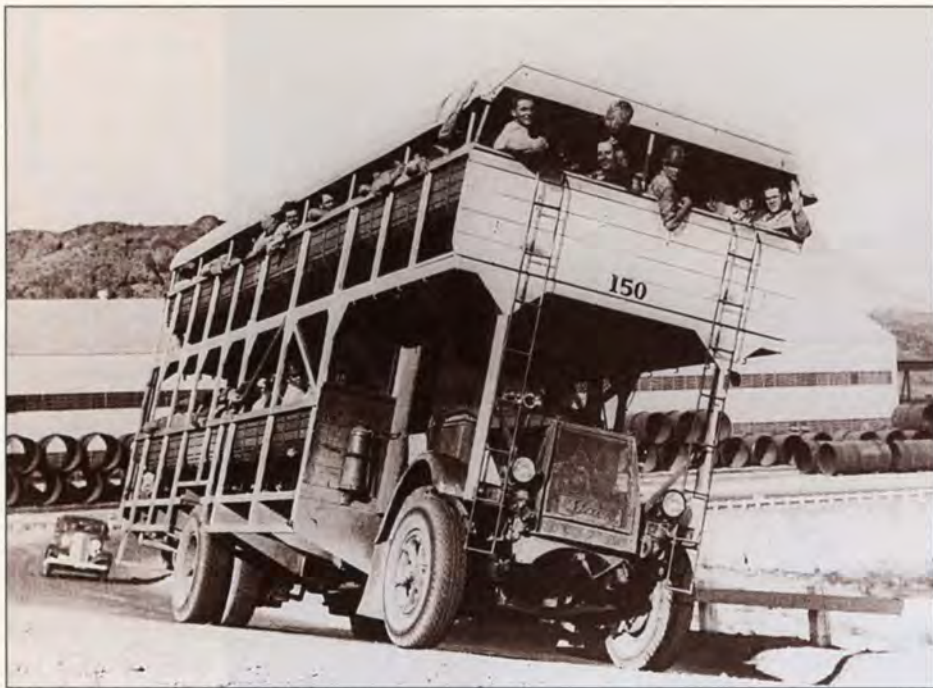
This Big Bertha transport bused 150 workers from Boulder City to the dam site.
