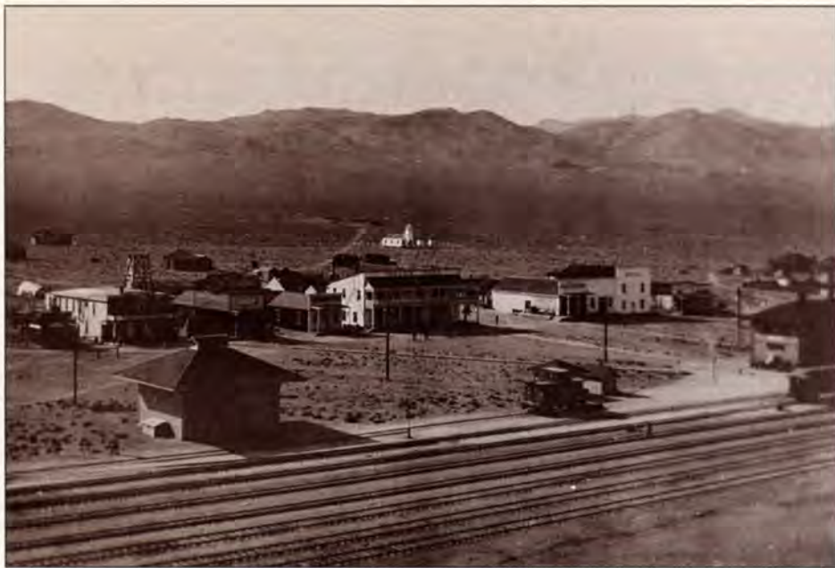
The railroad's water tower offered a panorama of Mina, named for Ferminia, about 1910.
