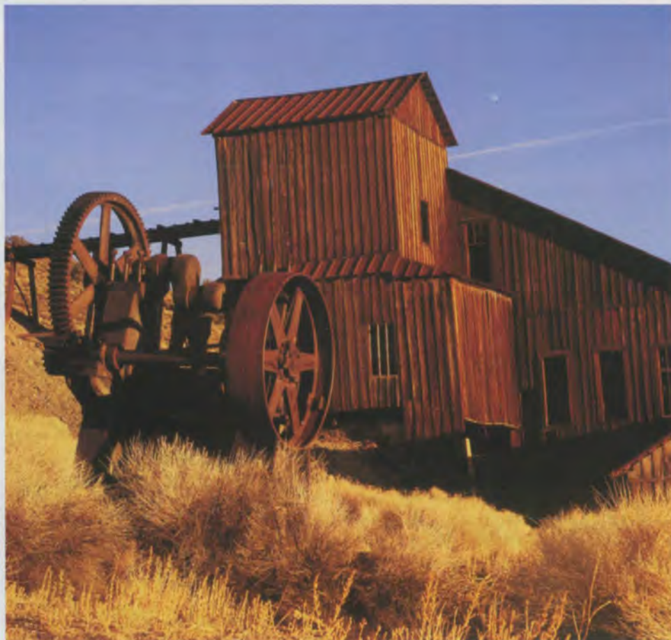
The 103-year-old Berlin Mill is one of 13 historic buildings still standing at Berlin-Ichthyosaur State Park.
