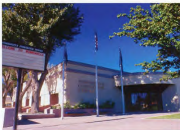
The Winnemucca Convention Center is a 32,000-square-foot complex.
