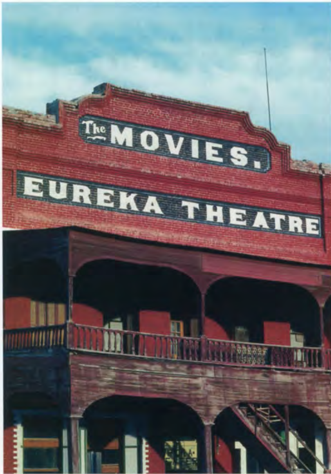
This photograph shows the Eureka Opera House before its restoration.
