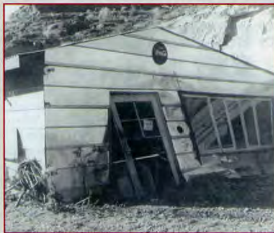
The Nelson’s Landing store was smashed by the 1974 flash flood. Nine people were killed, and cars and half the boat dock were swept into Lake Mohave.
