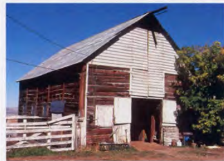
This historic barn in Lamoille will be on the Northeastern Nevada Museum tour.
