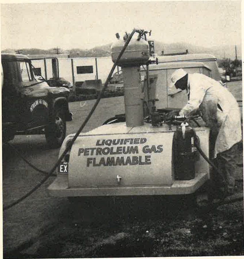
The inspection of liquid petroleum gas meters requires the use of special equipment and technical training.
